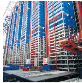
The modern high-bay warehouse ensures efficient logistics
